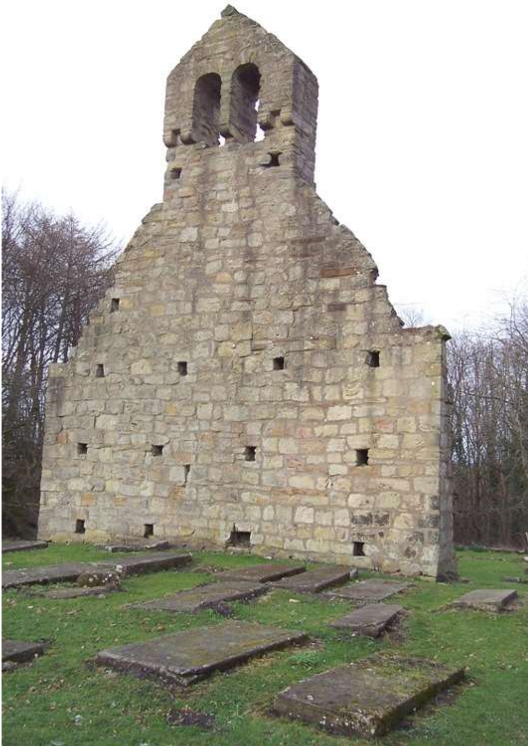
Illus 9: The remaining west gable.
